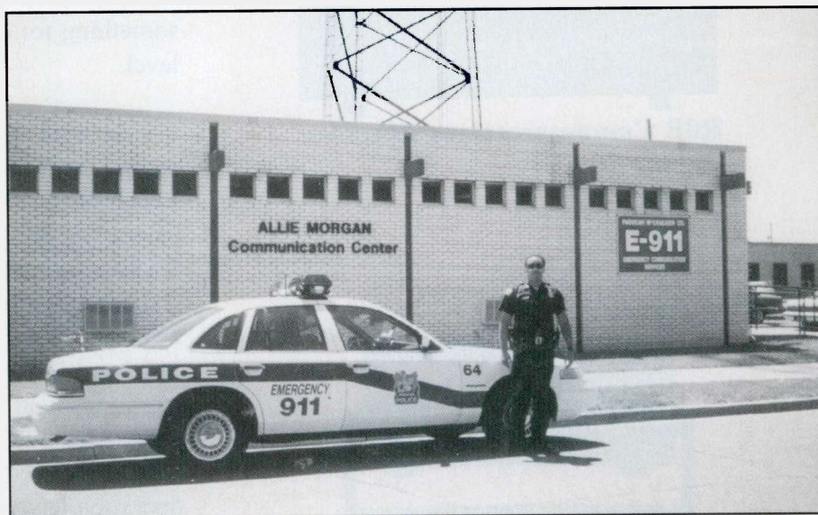
The author outside the Allie Morgan Communications Center. The center is home to McCracken County Central Dispatch which receives all 911 calls placed within McCracken County, and dispatches all the emergency agencies in the county including Paducah PD and Fire.
